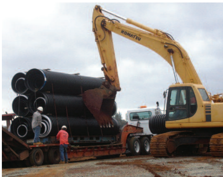
Melvin, Presley and Lorrin unloading drain pipes at Ka'iulani of Princeville
