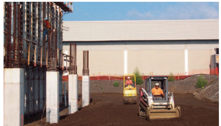
Brian Grace Jr. & Blane Ahsing backfilling at Hilo Judiciary Complex
