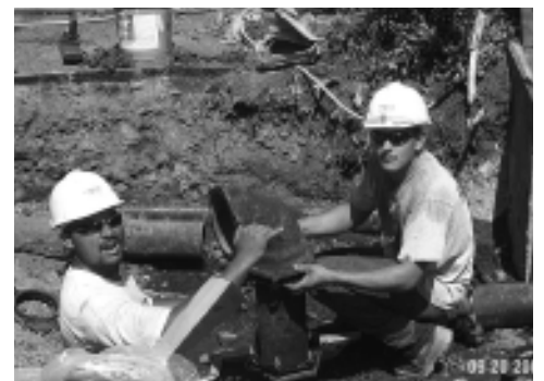
Guy & Blane - final water connections at Sheraton Keauhou.
