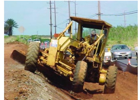
Derek Ebesu cutting slope at Kuhio Hwy. at S. Leho Drive
