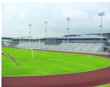
Kealakehe High School Increment 4 Phase II with Dick Pacific Construction.
