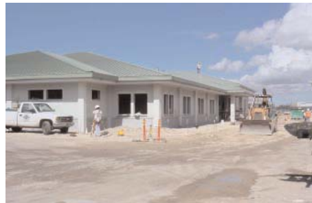
Department of Agriculture Annex 3 Project with Nordic Construction.
