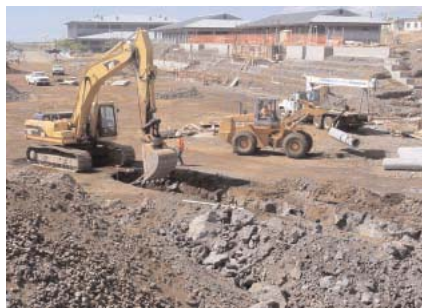
Kealakehe High School Increment 4 with Dick Pacific Construction.
