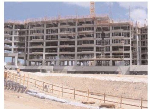
Marriott Ko Olina Timeshare Project with Dick Pacific Construction.
