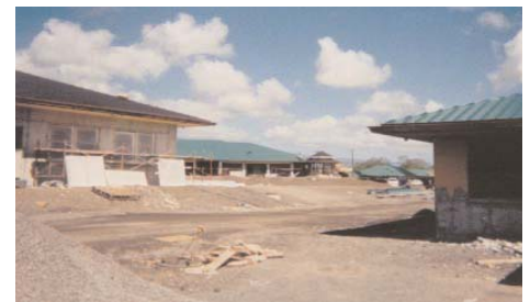
Kamehameha School East Hawaii Campus Phase 2 with Hawaiian Dredging & Construction Co.
