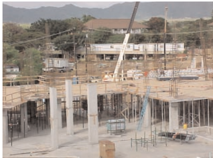
Work progresses at Marriott Waiohai
