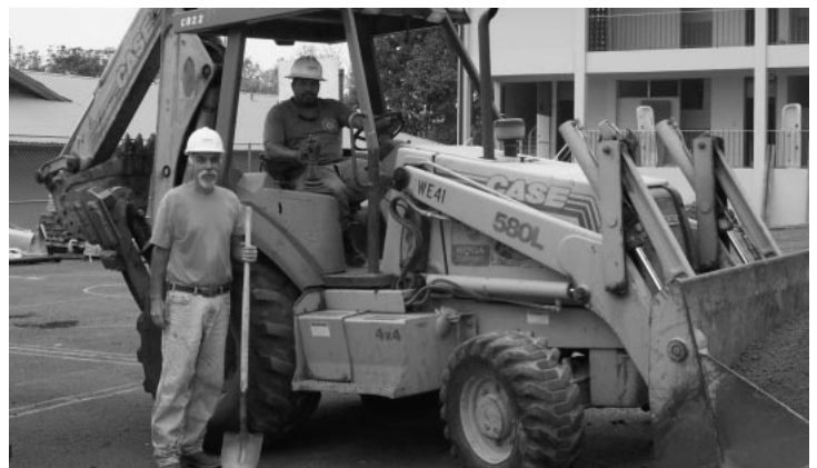
Irving & Rico at Konawaena Middle School Waterline.
