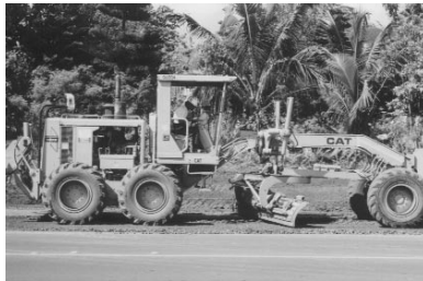
Derek "from Oahu" Ebese making the grade @ Miscellaneous Intersection Improvements.
